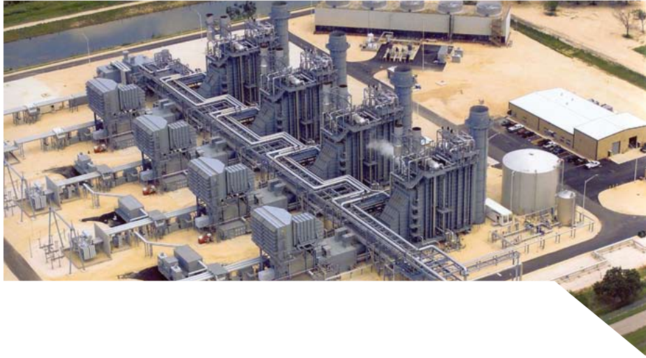
Channelview is an 800 megawatt natural gas-fired cogeneration facility in Texas that provides steam and electric power.
